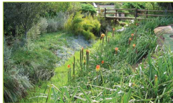
PERMEABLE STREAM LINING WITH COMPLETE PLANT COVER
