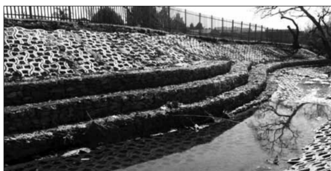
PERMEABLE HEAVY DUTY RIVER LINING
