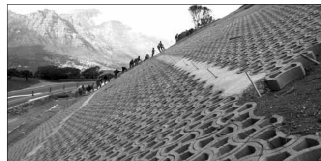
REINFORCED SLOPE STABILISATION
