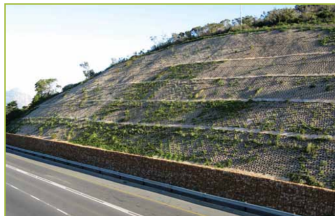
PERMEABLE SLOPE STABILISATION
