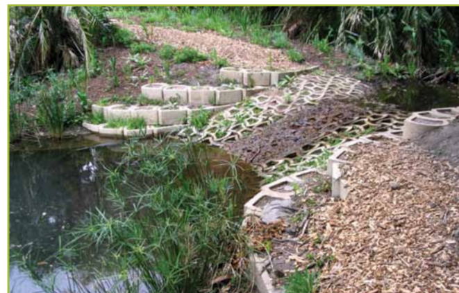
DAM SPILLWAYS AND INLETS
