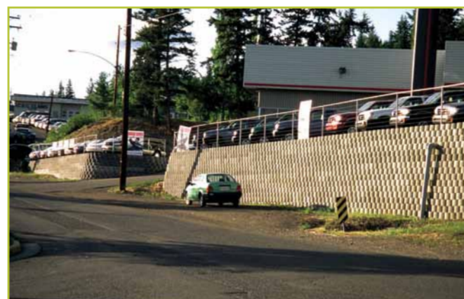
COMPOSITE WALLS IN ROUND FACE FINISH
