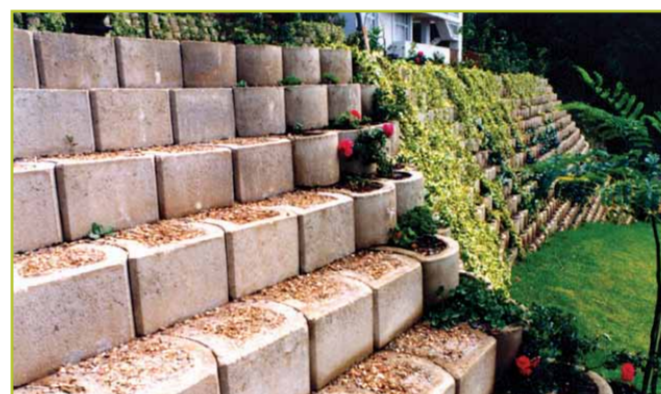
WALL AND STEPS, SMOOTH FACE FINISH
