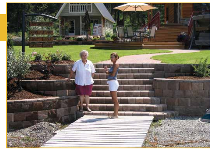
ACCESS STAIRS TO A LAKE WITH ROCK FACE RETAINING WALLS
