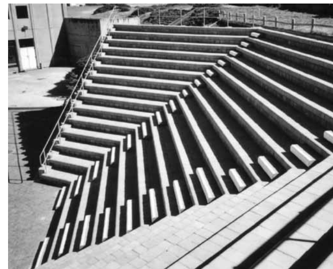
Seating arena and steps for 500 spectators
