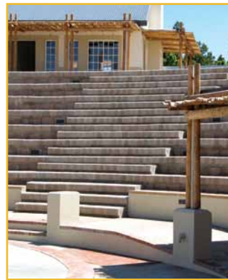
SEATING ARENA FACING STAGE
